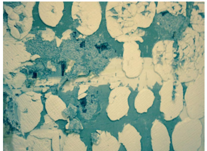
Spot bonding does not provide coverage as required under ANSI A108.5.
