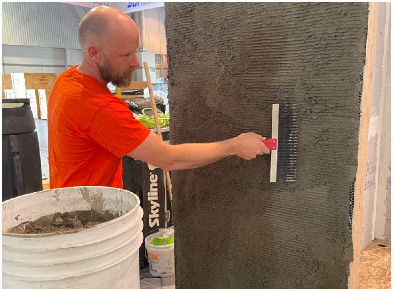
Thinset bond defective install. Photos courtesy of Dave Gobis.
