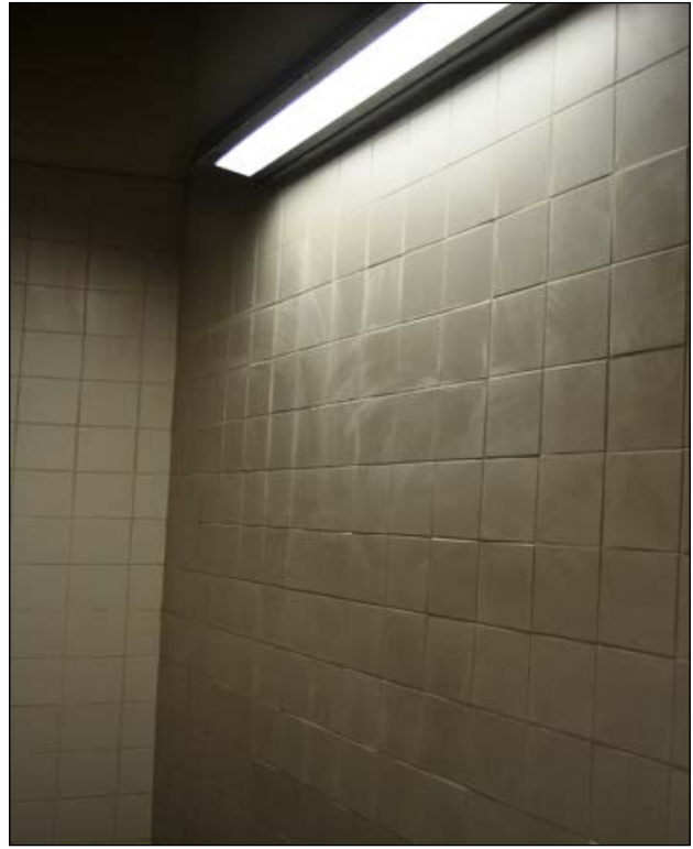
Light box, upward light, reflective ceiling can provide a softer more uniform profile to the tiled wall.
