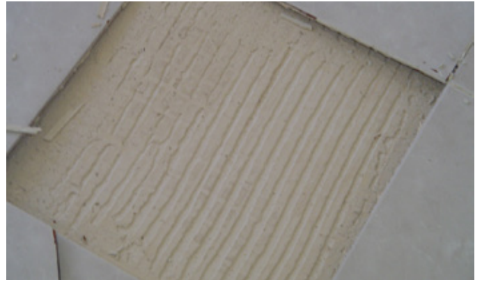
Thinset bond defective install. Photos courtesy of Dave Gobis.
