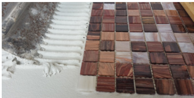
Photo #3 shows re-notching the previously flattened mortar to keep it fresh.
