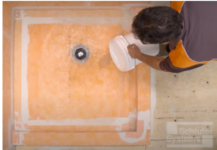
After installation perform flood test per manufacturer's written directions. Photo courtesy of Schlüter Systems.
