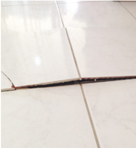
Lack of movement joints will cause pressure to build up and result in tenting of tile.
