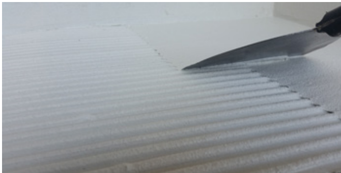
Photo #1 shows the ridges being knocked down with a broad knife.
