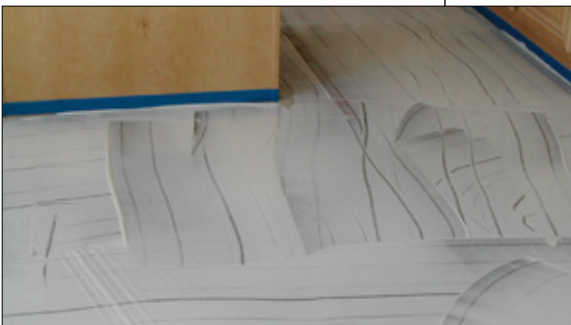
Using latexes other than those designed for the underlayment can act as a bond breaker.
