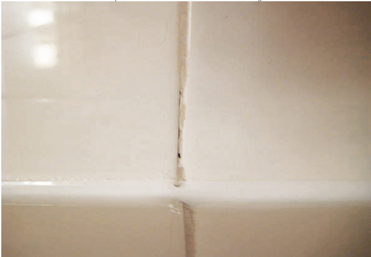
Pinholes in grout joints can result when the grout mix is too wet.
