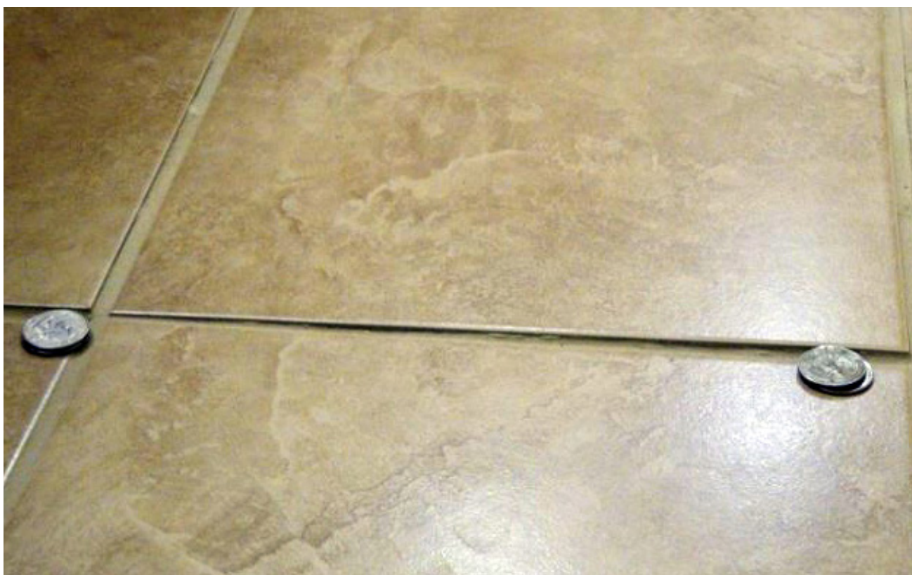
Variation in the height of adjoining tiles is called lippage. This is defined in the ANSI (American National Standards Institute) standard A108.02, Section 4.3.7: "Lippage refers to differences in elevation between edges of adjacent tile modules."
