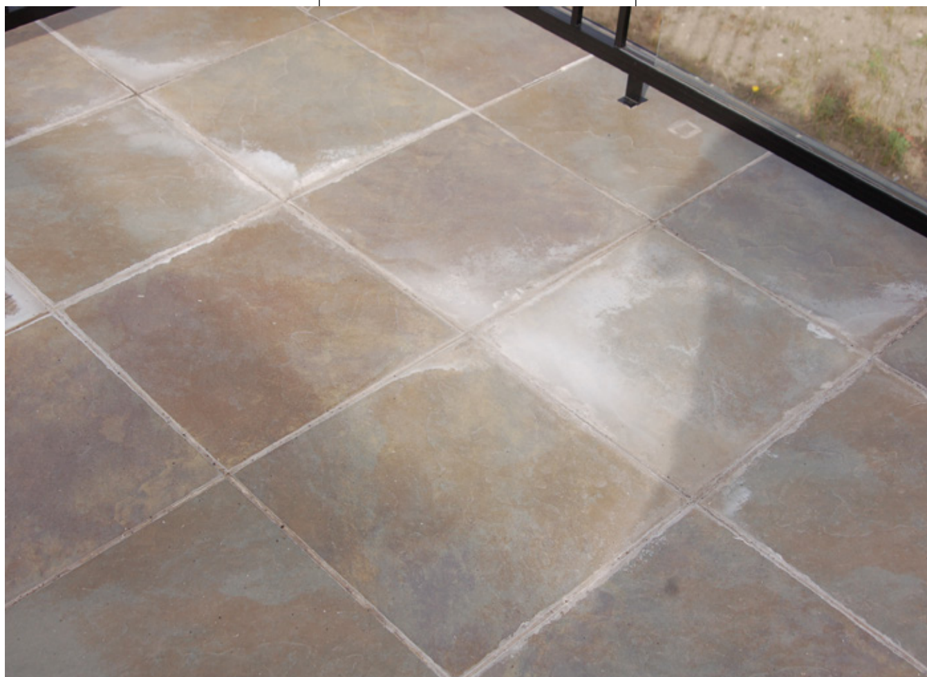
Efflorescence is seen here due to an uncured slab. Photo courtesy of Dave Gobis.
